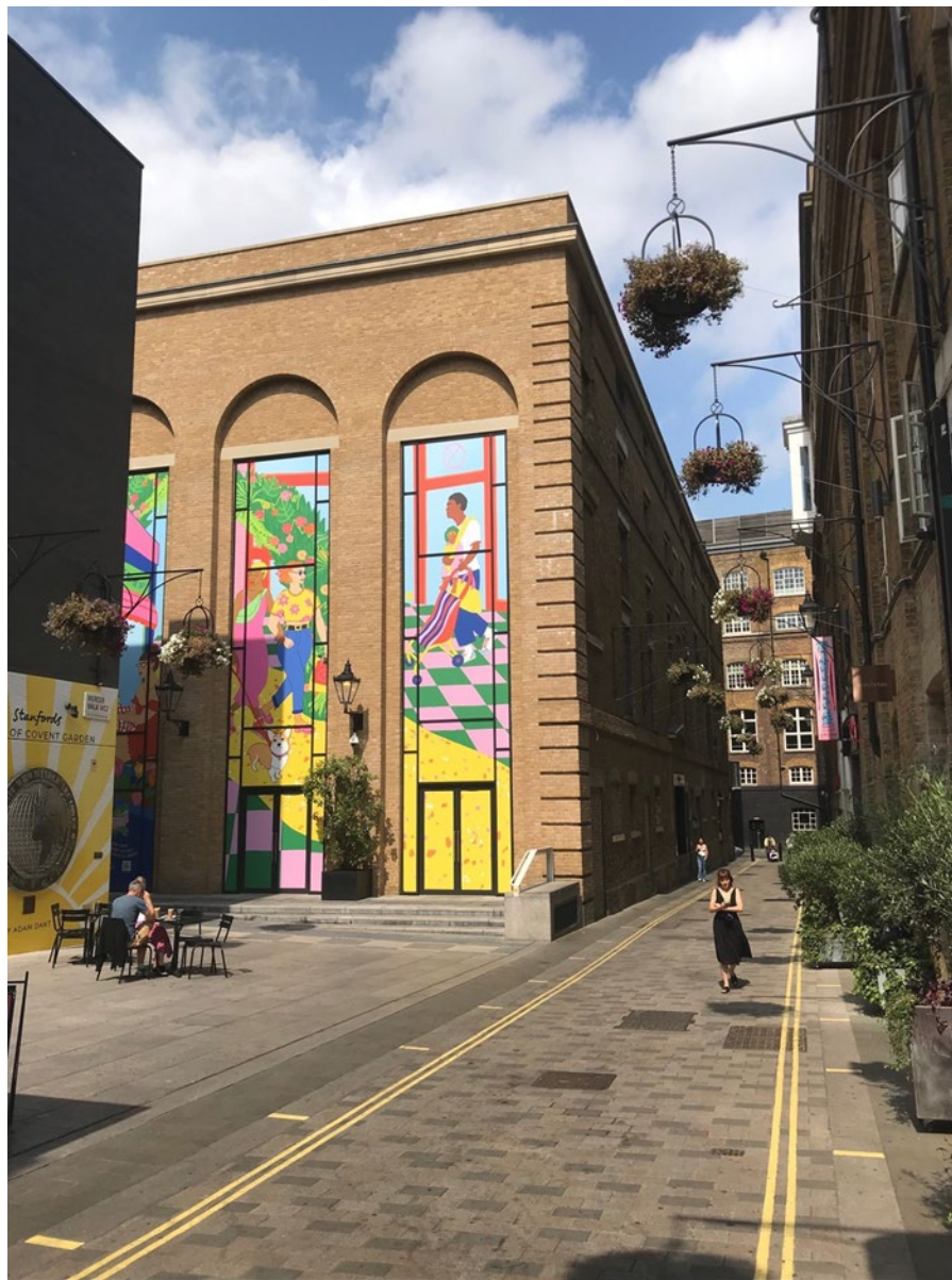
1 Mercer Walk, Langley Street
