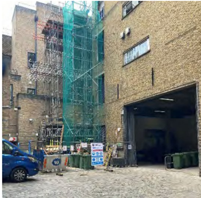
REAR OF 7 LANGLEY STREET (EXISTING)
