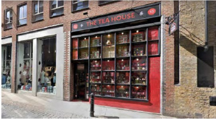
15A, Neal Street – Existing West Façade
